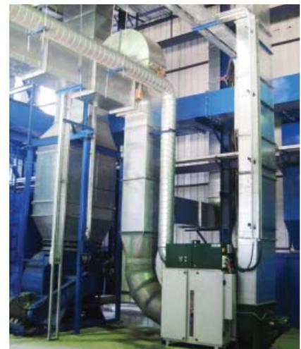
**The dehumidifier system is integrated into the Blasttechnik TDF ventilation dust collector. A variety of dehumidifying modes are selectable depending on the requirement.**
